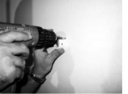
Move unit away from wall and remove Wall Flange from Tube and mount Flange to wall using 12 #10 x 1-1/4" Wall Mount Flange Screws (**#3**) and Plastic Wall Anchors (**#4**) if needed.
