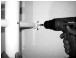
Slide unit back against wall while inserting all 4 Wallmount Extension Tubes (**#7**) into Wallmount Flanges (**#6**) and fasten with 4 - #08 x 3/4 Fastening Screws (**#1**).
