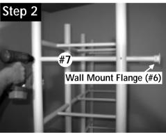
Move unit away from wall and insert 4 Wall Mount Extension Tubes (**#7**) at 4 Locations. Fasten With 8 - #08 x 1-1/2" Extension Tube Fastening Screws (**#2**) **Note: 1 Fastener Per Joint Front Side Only**
