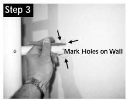
Slide Wall Mount Flanges (#6) into Wall Mount Tubes (#7) Place unit against wall where it is to be mounted and mark Wall Flange holes. Note: Do NOT fasten at this time. Make sure unit remains in position at all 4 locations while marking holes.
