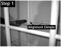
Fasten all Verticals to Horizontals. Make sure all joints are pressed firmly together, tight and against alignment dimples. 32 - #08 x 3/4" Fastening Screws (#1) *Note: 1 Fastener Per Joint, each grid, Front Side Only*
