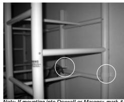
Note: If mounting into Drywall or Masonry, mark & drill 1/4" holes and insert plastic wall anchors - and proceed with step 1-
