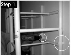
Place 4 wallmount brackets (**#6**) over 4 Rear Verticals above 2nd Horizontal Crossbar (**#1**) and fasten to wall using 8 - #10 x 1-1/4" Fastening Screws (**#2**)
