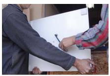
Once the base is in position, insert the two 1/2-13 flat head socket screws and tighten using a 5/16" hex key.
