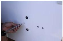
Insert the three wood screws and tighten them.
