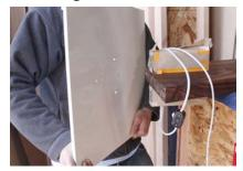
This step should be performed by two people due to the weight of the base. One person should hold it in position while the other inserts the fasteners.
