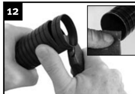
Cut the tube at the groove using a sharp utility knife to ensure a square, flat cut. Clean burrs from the cut end with emery paper.
