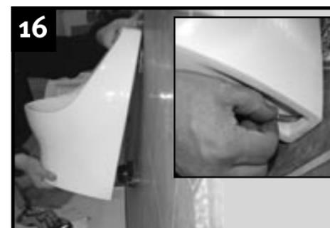
Hang the bowl, inserting tailpipe into bushing, then install anchor screws with washers. Tighten flange bolts and gear clamp.
