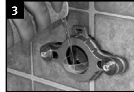
Clean face of existing wall flange then install the brass flange with the clear inspection disc. Slowly pour water into the drain.
