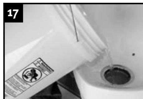
Pour 5 gallons of water as rapidly as possible into housing to ensure good flow and no leaks or standing water.
