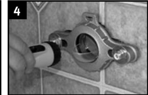
Use a flashlight to check pitch/slope. There should be no water present in the inspection disc or nipple. Remove flange after inspection.
