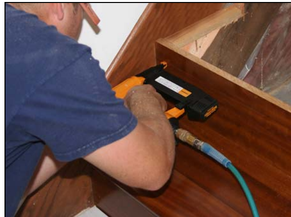
Nail the riser face into the stringer.
