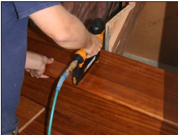
Nail from the tread into the stringer.
