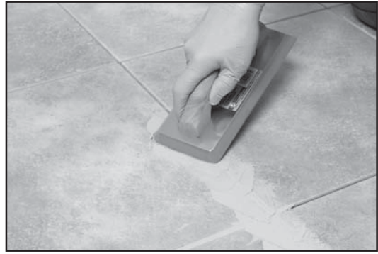
Fig. 21 - Pack the grout into the joints.
