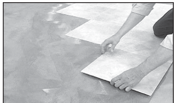
Fig. 15 - Install ungrouted floors following a stair-step pattern.
