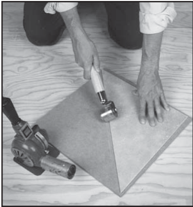
Fig. 20 - Roll the cut edge to form a slight radius.
