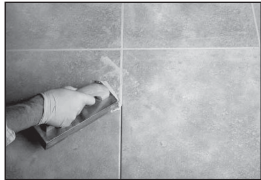
Fig. 22 - Extend grout a few inches into the next row.
