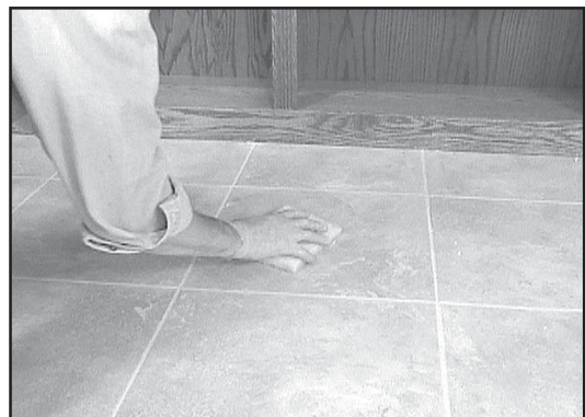
Fig. 23 - Use a 3M white, nylon pad to loosen grout residue.
