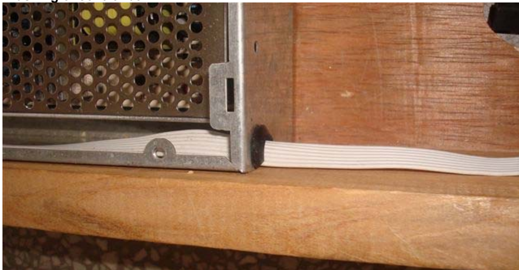
Photo 40 - Bushing of control box
