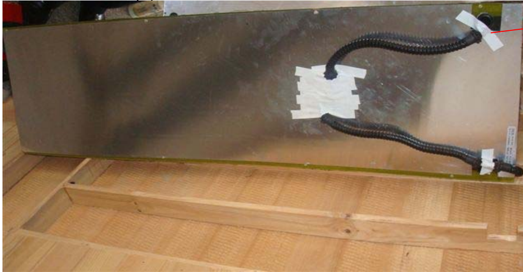
Photo 49 - Back view of Heater (III)
