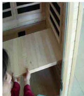
FIG-10 Assembling bench
