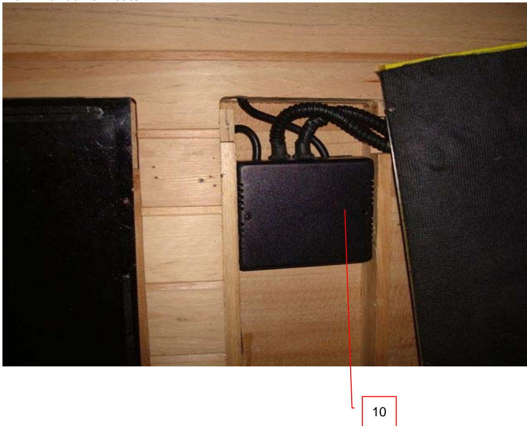
Photo 46 - Terminal box of heater
