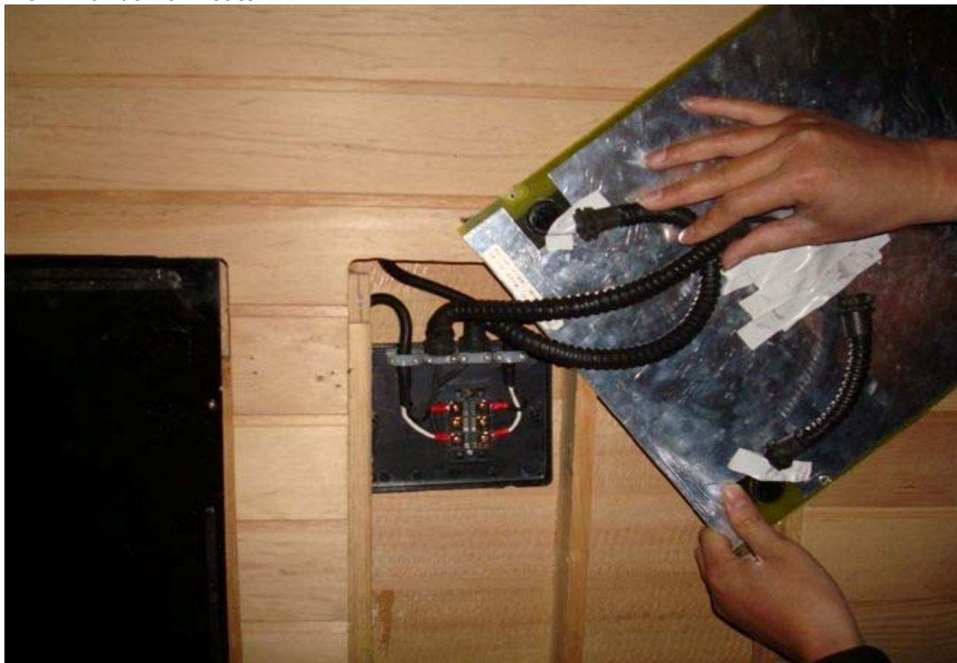
Photo 54 - Terminal box of Heater
