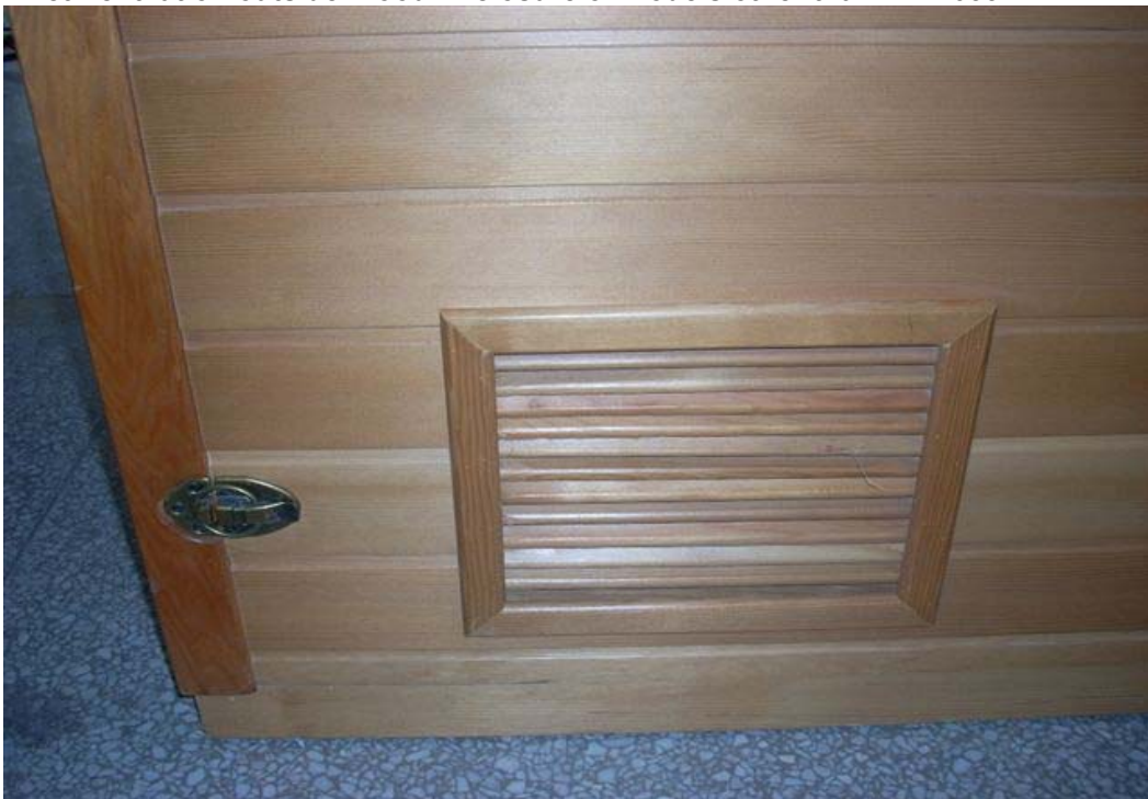
Photo 26 - Inlet Ventilation outside Wood Enclosure of models other than FRB-033LWT
