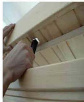
FIG-14 Leading the wires of heaters onto the board through the corresponding hole
