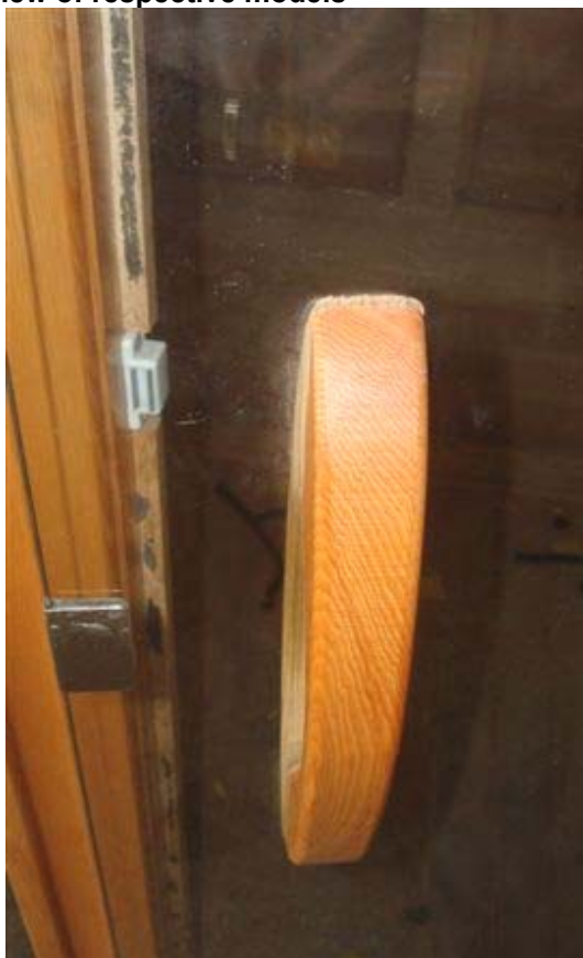
Photo 21 - Wood handle and Magnetic catcher provided for all models. See detailed shape in photos of external view of respective models
