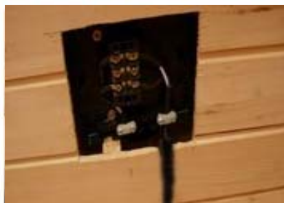
FIG-9 Connecting wire
