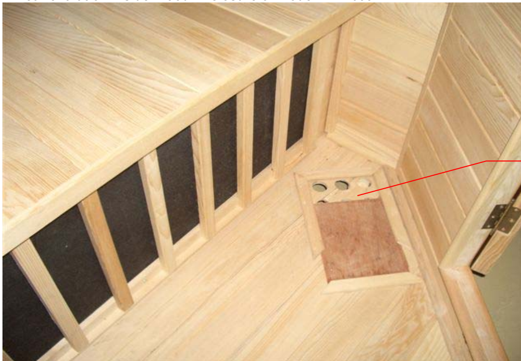
Photo 28 - Inlet Ventilation inside Wood Enclosure of model FRB-033LWT
