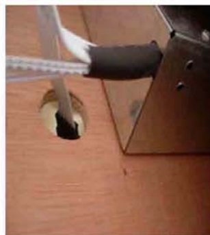
FIG-16 Put down the wires into the sauna cabin
