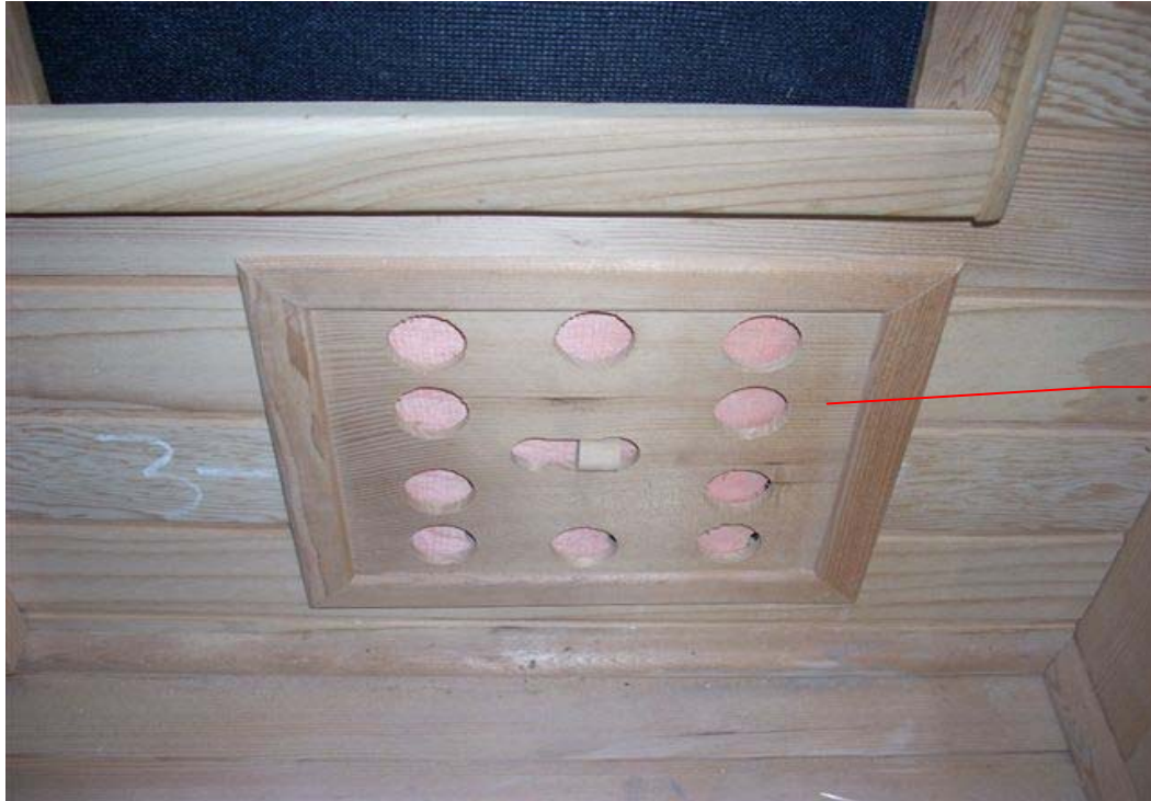
Photo 27 - Inlet Ventilation inside Wood Enclosure of models other than FRB-033LWT
