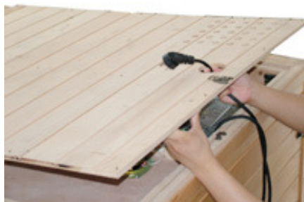
FIG-19 Slip the power plug through external top board
