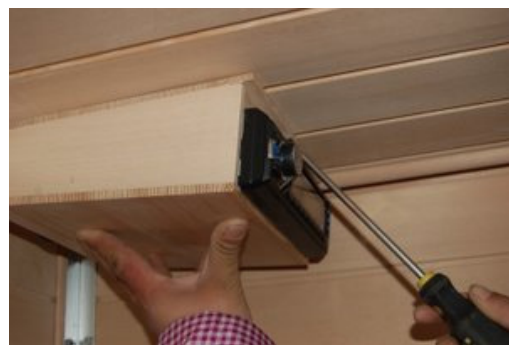
FIG-18 Fix the CD player back cover with screws
