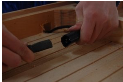
FIG-14 put down the wires into the sauna cabin
