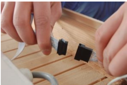
FIG-13 Connectors on the internal top board
