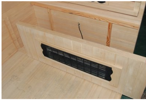
FIG-7 Assembling bench chair bracket
