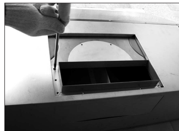
E. Mounting rectangular starting collar with remaining screws.
