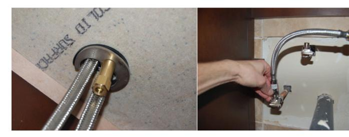
The two photos below show a different installation using a different <u>vessel sink faucet</u> that has a lock nut mount, which screws to a threaded piece of pipe attached of the body of the faucet. The photo on the left show the connection of the supply lines, the photo on the right shows the tightening of the nut to affix the faucet to the countertop. Once the faucet is mounted, the same process of connecting the supply lines to the threaded connector on the water supply pipes would apply.
