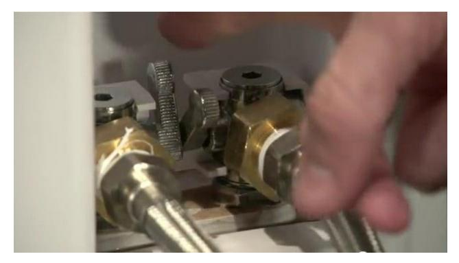
Before mounting the shower panel, connect the hot & cold waterline to test for any leaks. if there is leaks at back of the clamps, you can fix the clamp with screw driver & clamps.
