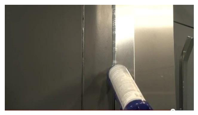
finally, run the silicon at left & right of the panel, but not the bottom; this allows any possible future leaks to drained rather get trapped in the wall.
