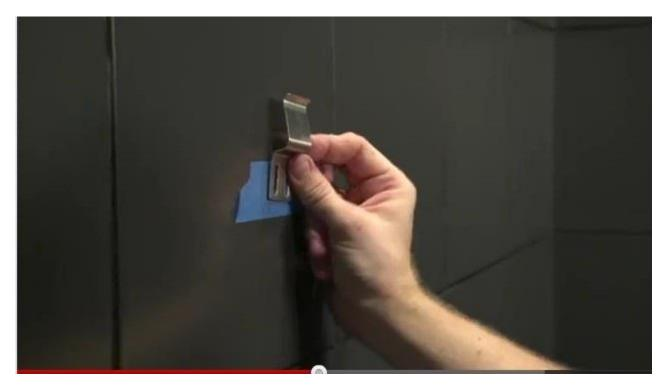
Measure and attach 2 brackets onto wall. make sure the hose will reach the shower pipe from your mounting location.
