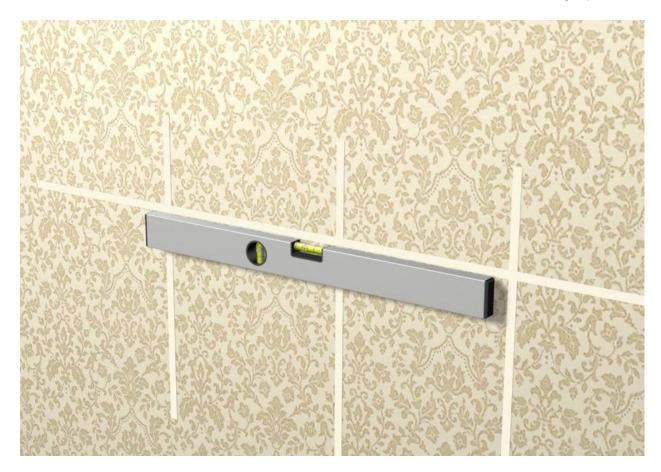
Place a level where the shelf is to be located and mark again with masking tape.
