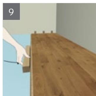
**10.** When three rows have been laid, the distance from the floor to the walls can be adjusted. Place wedges between the floor and wall.
