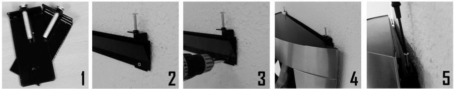
The "safety bracket" (1) is to mount together with the wall bracket as shown in the pictures (2 & 3). It comes in the back of the wall bracket. Hang the fireplace on the wall bracket (4) and then tightened the screws of the "safety bracket" (5). Make sure that the fireplace does not move anymore.
