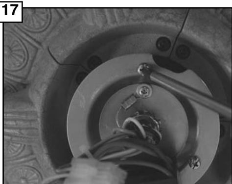
Remove 1 screw and save. Loosen other 2 screws.
