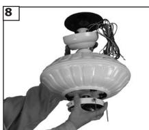
Carefully lift fan assembly onto mounting bracket. Rotate fan so that the notch on the ball engages the ridge in the mounting bracket. This will allow hands-free wiring.
