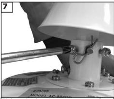
Tighten both yoke set screws to further secure downrod.
