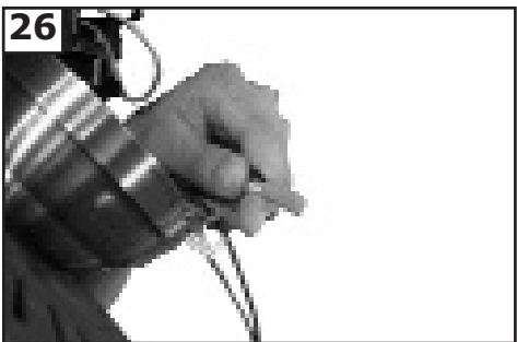
26 Make wire connections to power source using wire nuts provided. Make sure that no filaments are outside of the wirenut. After making the wire connections, the wires should be spread apart with the grounded conductor and the equipment-grounding conductor on one side of the outlet box and ungrounded conductor on the other side of the outlet box.
