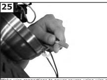
Make wire connections to power source using wire nuts provided. Make sure that no filiments are outside of the wirenut. After making the wire connections, the wires should be spread apart with the grounded conductor and the equipment-grounding conductor on one side of the outlet box and ungrounded conductor on the other side of the outlet box.
