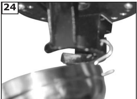
Hang fan from mounting bracket by the hands free "S" hook in hardware pack into a closed hole on the edge of the canopy and over bracket..
