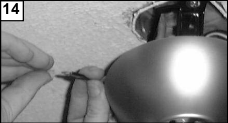
14 Make wire connections to power source using wire nuts provided. Make sure that no filaments are outside of the wirenut. After making the wire connections, the wires should be spread apart with the grounded conductor and the equipment-grounding conductor on one side of the outlet box and ungrounded conductor on the other side of the outlet box.
