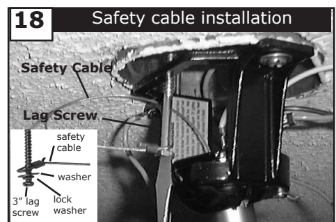
18 Safety cable installation Safety Cable Lag Screw safety cable washer lock washer 3" lag screw For Canadian installation and for USA fan and light kit combinations over 35 lbs, in both flush and downrod mode the safety cable must be installed into the house structure using the 3" lag screws, washers, and lock washers provided. Make sure that when the safety cable is fully extended the leadwires are longer than the cable and no stress is placed on the leadwires.
