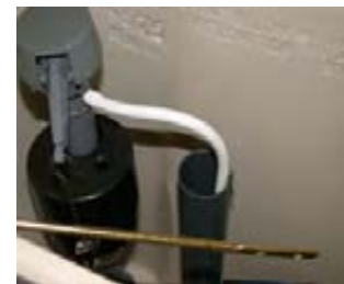
Alternate view of the refill tube attachment.
