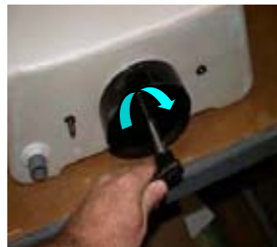
Tighten the lock nut hand tight plus an additional 3/4 turn.
