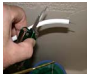
Remove 2 inches (50mm) from the end of the refill tube; save the "S" clip for the next step.
