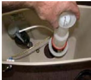
Remove the old flush tower and discard.
