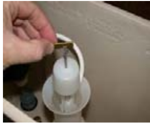
Sponge out any remaining water. Detach the hook from lift arm.
