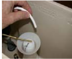
Disconnect the refill tube from the tower. Detach the tank from bowl by removing tank fasteners. (not shown)
