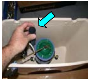
Install a New Champion4 Flush valve with the vent tube positioned as shown.
