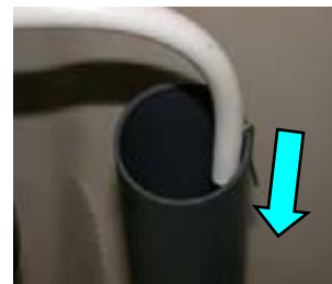
Affix the end of the refill tube to the valve overflow at the location shown.
