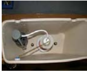
Turn off and disconnect the supply line. Drain the tank by lifting tower.
