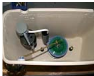
Properly configured Champion4 Flushing System.
