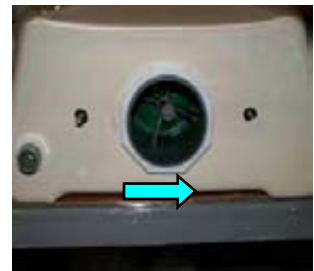
Align the lock nut "flat" parallel to back edge of tank.
