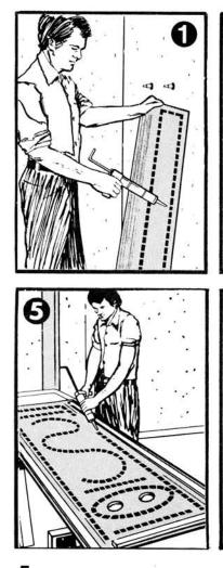
**5** Apply adhesive to proper side panel with pattern suggested. Keep adhesive 1" away from factory applied pressure sensitive tape. Put extra ring of adhesive round drilled holes. **2** Remove backing from factory applied pressure sensitive tape.
