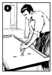
**4.** Use a drill with a hole cutting bit, or a hole saw to cut the openings for the faucet and handle outlets. Cut the holes 1/2" larger than the diameter of the outlets.
