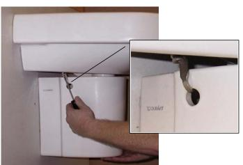
b) Insert the hooks into the holes on the sides of the siphon cover. Using your fingers or a phillips screwdriver, tighten the screw until the siphon cover is secure under the washbasin. Do not over tighten!
